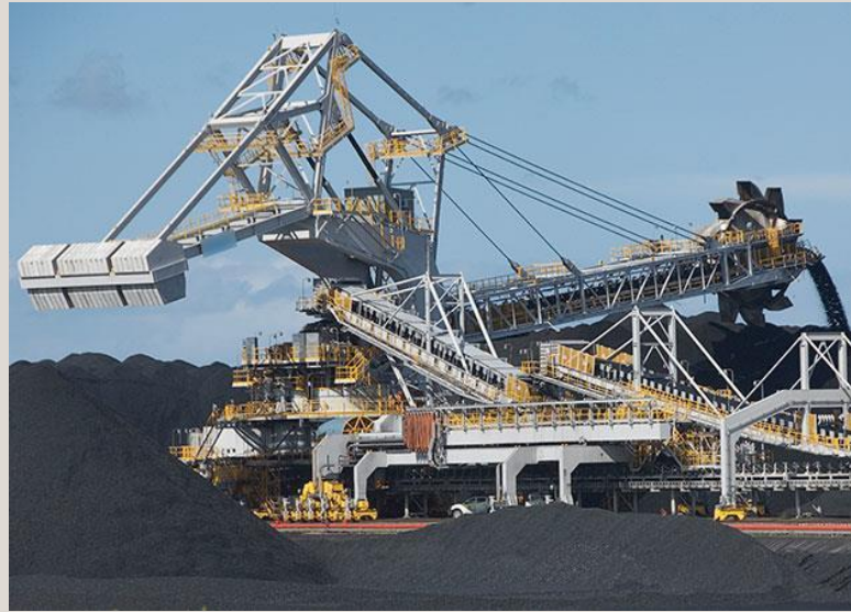
NCIG Coal Export Terminal (Newcastle, NSW, Australia - 2011-2013)
