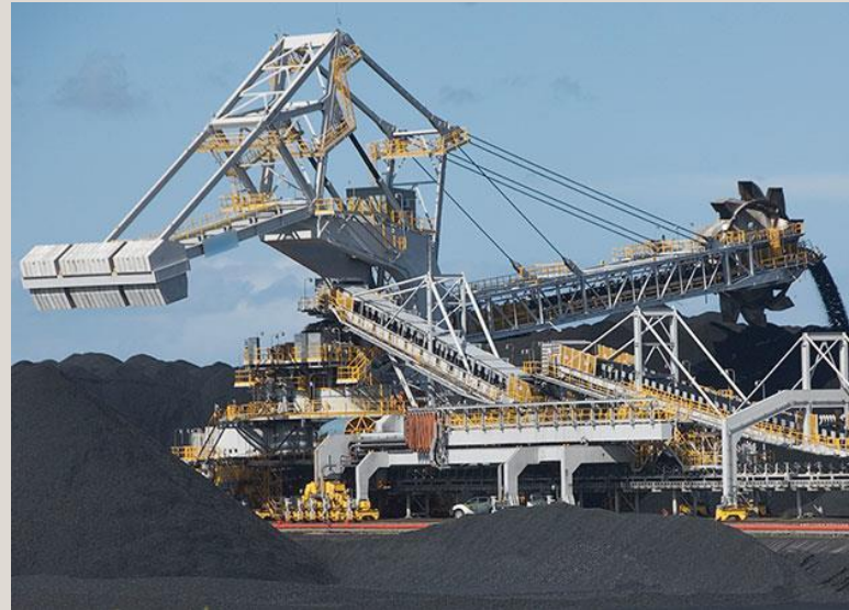
NCIG Coal Export Terminal (Newcastle, NSW, Australia - 2011-2013)
